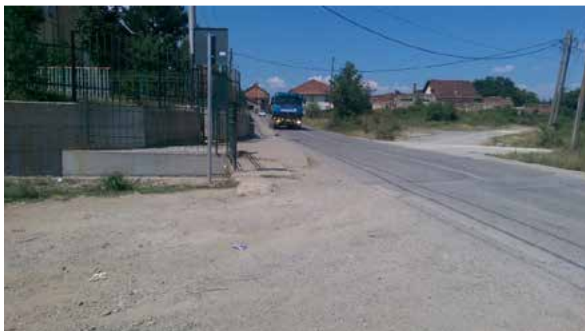
Fig. 5. Lack of signaling
