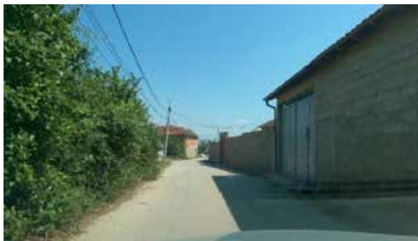
Fig.9. Lack of signaling
