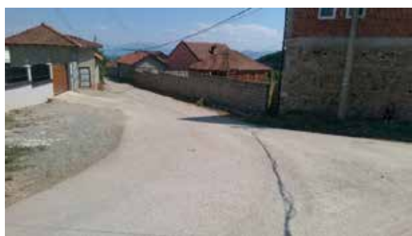
Fig. 7. Lack of signaling
